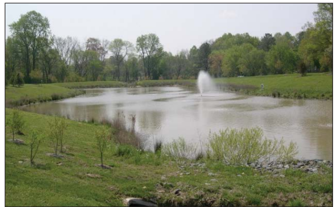
Stormwater ponds, like this one in Easton, Maryland, capture runoff and reduce nutrients in the water.
